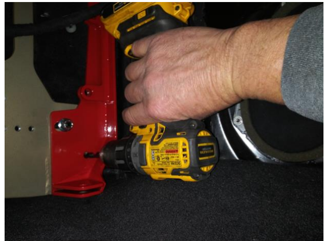
Fig. 11 - drilling holes for M8 stud plates
