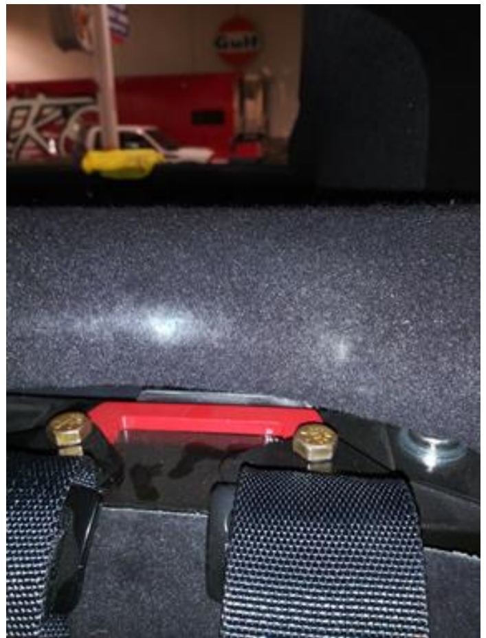
Fig. 16C - red spacer plate and shoulder belt installed 7/16-20 bolts are used to install shoulder belts, use Loctite blue 242 on all belt mounting bolts
