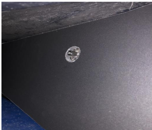
Longer side of the peel rivet through the stake
